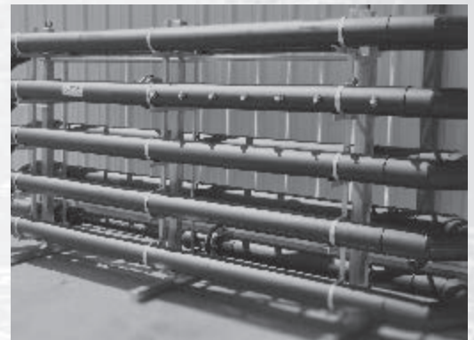
AIR INJECTORS DISSOLVED AIR ENTRAINER'S
